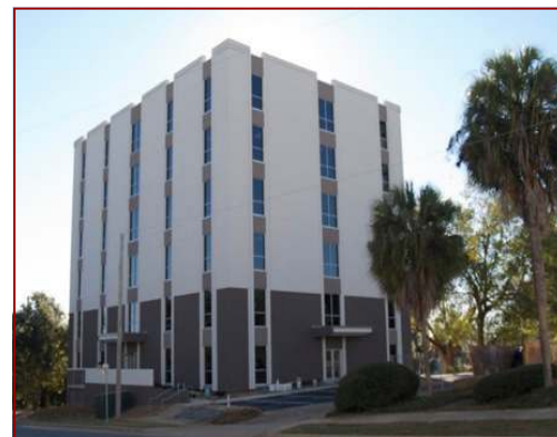
New SCSD Building—Warren Building
